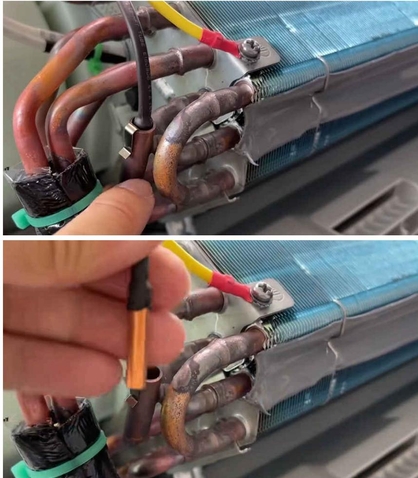
**Figure 1-2. Position of the Temperature Sensor for Evaporator Coil**
