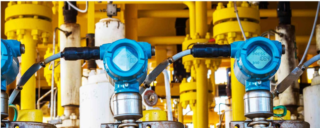
**Figure 1. Pressure Transmitters**
